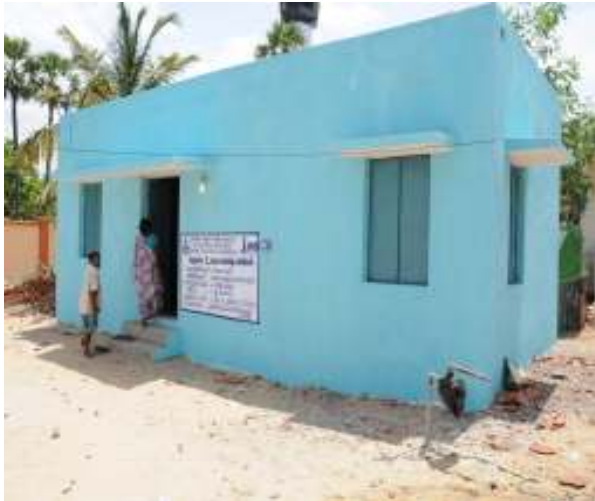
FMS Building, Thiruvallur District.
